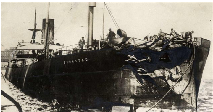
Below: The Storstad's damaged bow.
